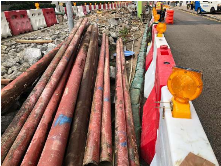
Figure A5: Sandbags were provided along the site boundary for site in Ching Ping Street
