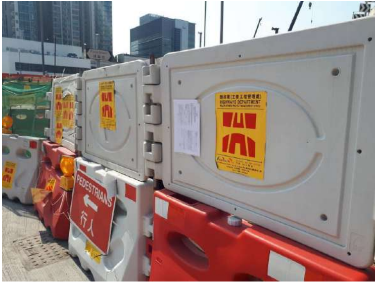
Figure A2-4: Posting CNP at the entrance and on hoarding of Zone B2
